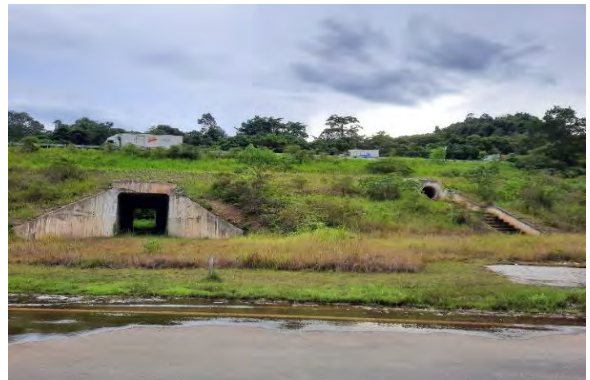
Box Culvert C-PL1
