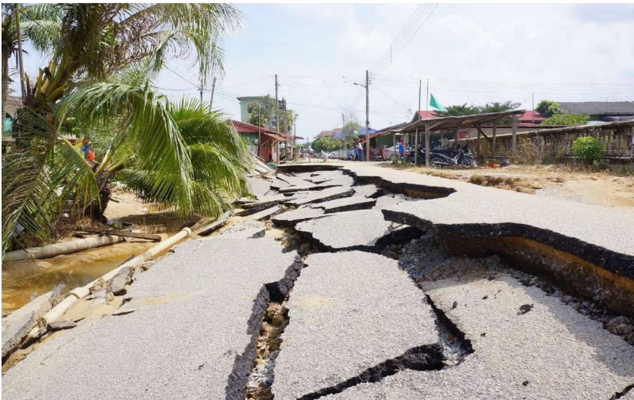
Damaged road due to flood in Kg Tanjung Kuala, Tumpat, Kelantan.
