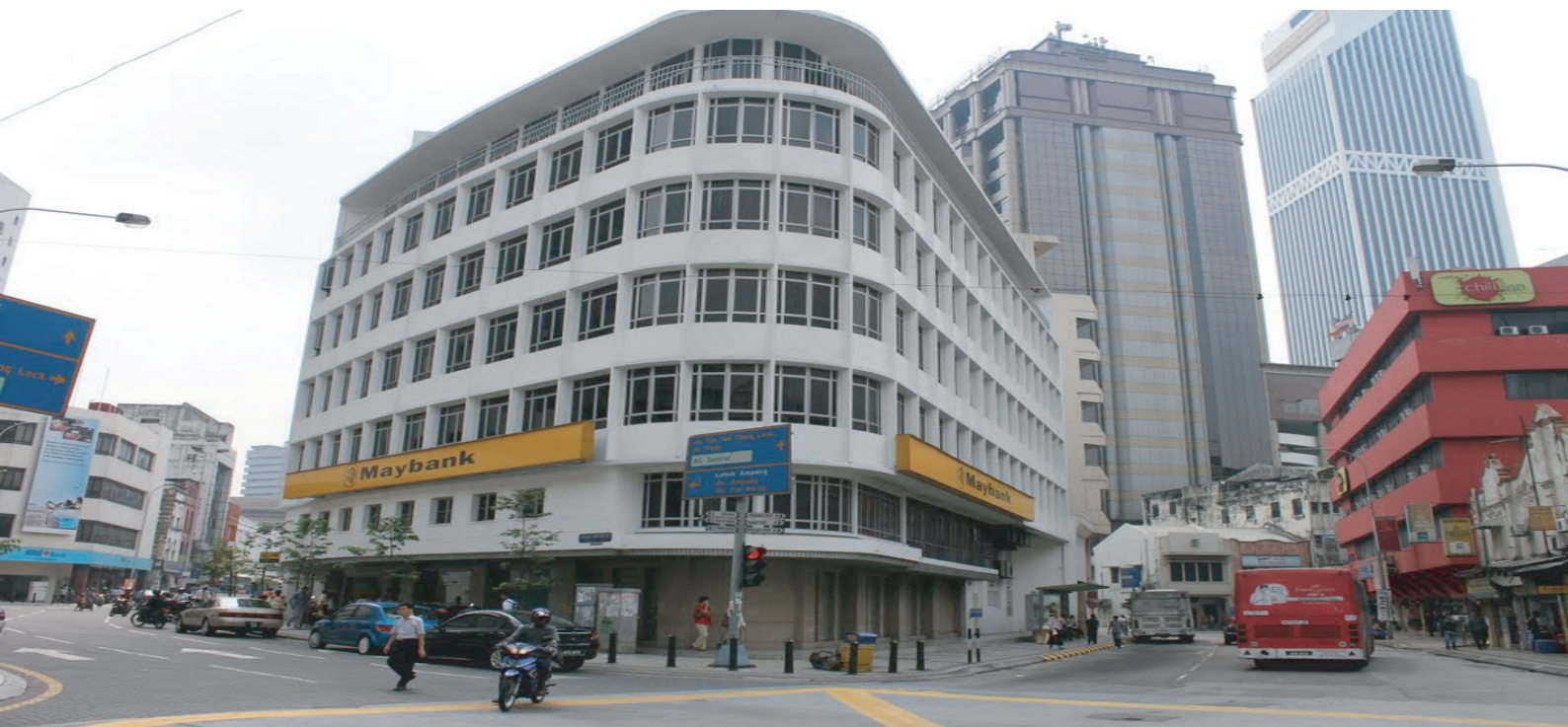
Maybank, Jalan Tun H.S Lee
