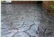
Laluan Pejalan kaki (concrete imprint)
