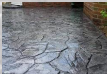
Laluan Pejalan kaki (concrete imprint)
