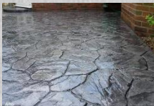
Laluan Pejalan kaki (concrete imprint)
