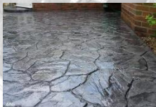
Laluan Pejalan kaki (concrete imprint)
