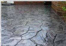
Laluan Pejalan kaki (concrete imprint)
