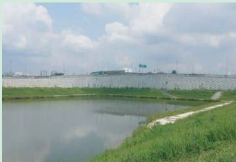
Kolam takungan banjir Puah, Selangor
