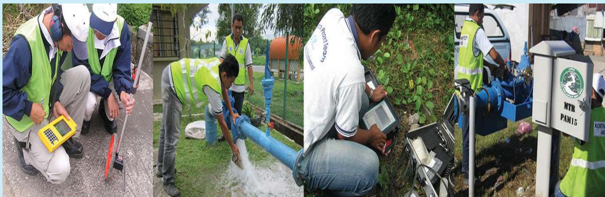
Examination and replacement of old pipes are being undertaken
