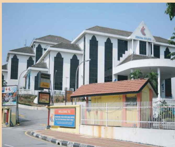
Kuala Lumpur International Youth Centre located in Bandar Tun Razak, Cheras
