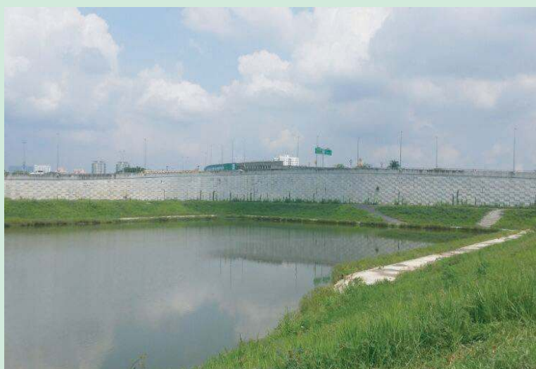
Flood pondage area in Puah, Selangor
