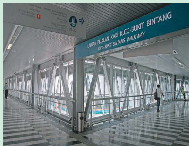
Covered walkway connecting the Kuala Lumpur Convention Centre (KLCC) with Bukit Bintang
