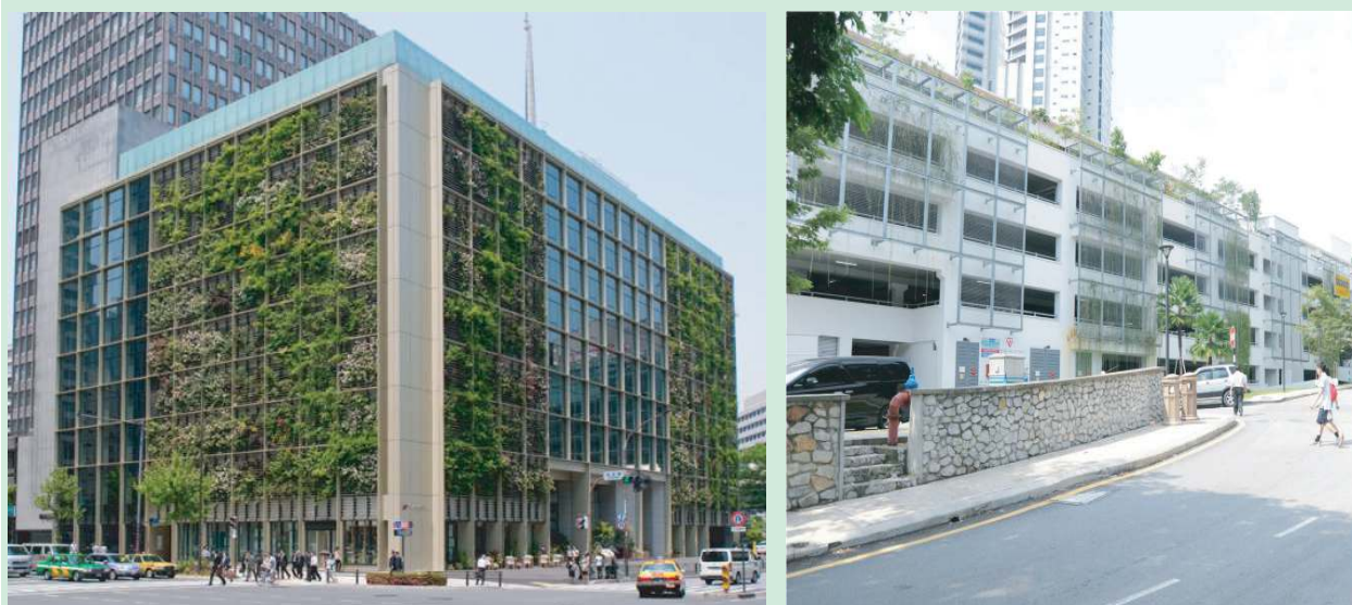
The provision of green areas on buildings can help reduce carbon emission and urban heat island intensity
