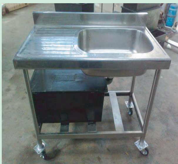
Grease traps installed at food premises
