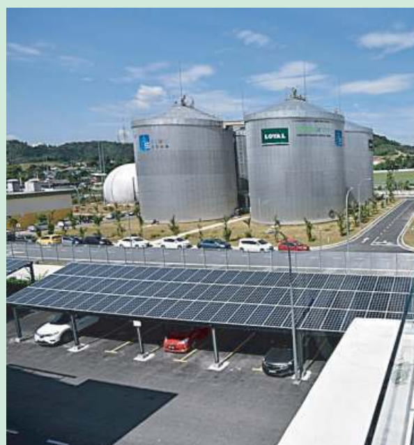
The Pantai 2 sewerage treatment plant, located in Pantai Dalam, Kuala Lumpur is the largest in Malaysia
