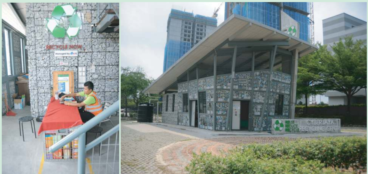
Collection centre for recyclables provided in Cyberjaya
