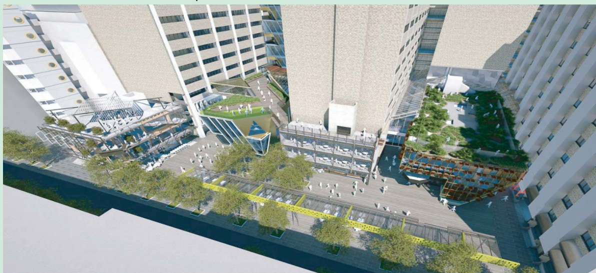
The New Academic Street RMIT University which retrofitted the buildings themselves
