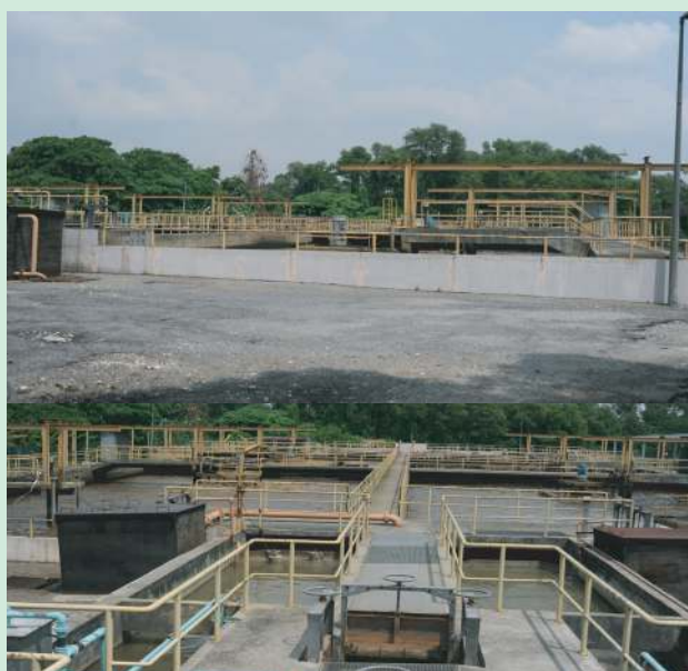
Sewerage treatment plant located in Hulu Langat
