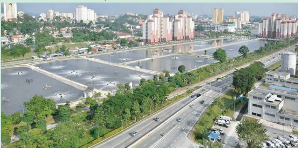
The Pantai 2 Sewerage Treatment Plant in Federal Territory Kuala Lumpur is a new innovative project to upgrade open treatment plants to a closed underground one complete with public services.
