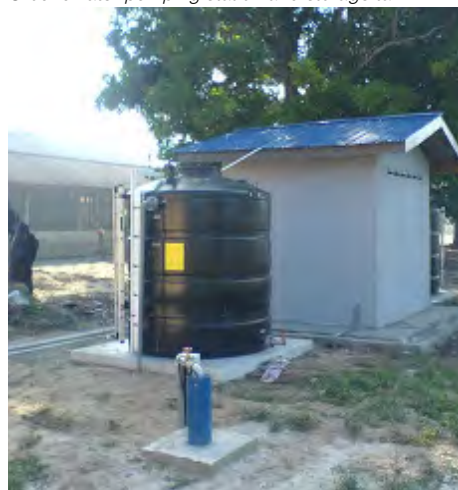
Groundwater pumping station and storage tank
